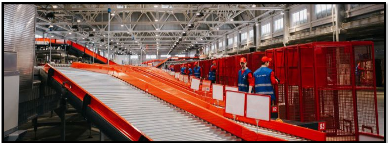
Figure 1 – «Nova Poshta» Kyiv Innovative Terminal
